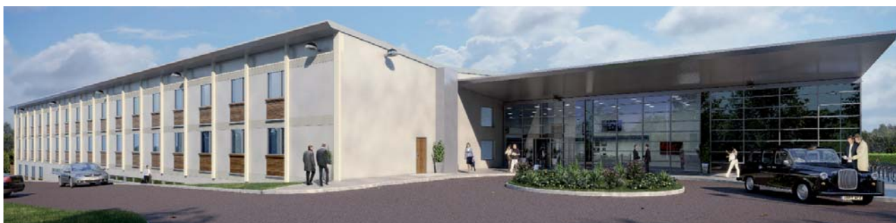
The Holiday Inn hotel in Winchester, being built by Bond Contracting Limited.
