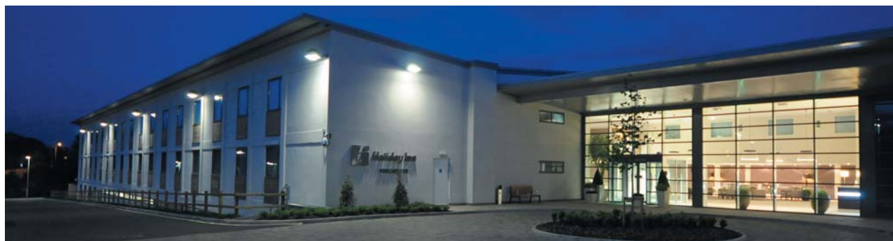
The Holiday Inn Hotel in Winchester, built by Bond Contracting Limited.
