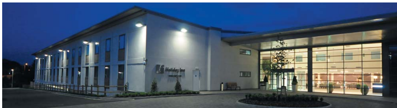
The Holiday Inn hotel in Winchester, being built by Bond Contracting Limited.
