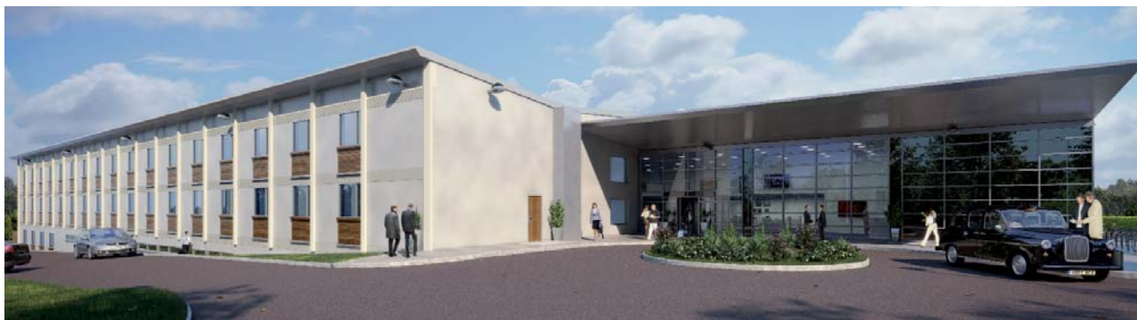
The Holiday Inn hotel in Winchester, being built by Bond Contracting Limited.
