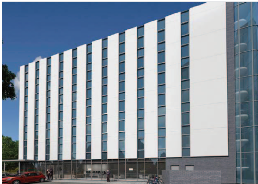
CGI of 134 bedroom Ibis Budget Hotel currently under construction
